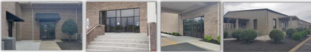
Worship Center near Restrooms
