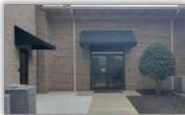
Worship Center near Restrooms
