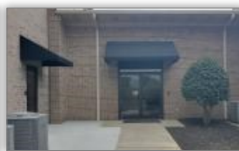
Worship Center near Restrooms
