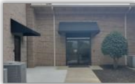
Worship Center near Restrooms
