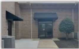
Worship Center near Restrooms
