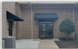
Worship Center near Restrooms
